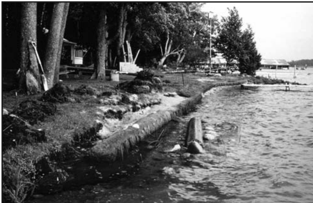
Figure 28: Coir staked in place, with sod excavation and stockpiling, and sand backfilling in progress.
