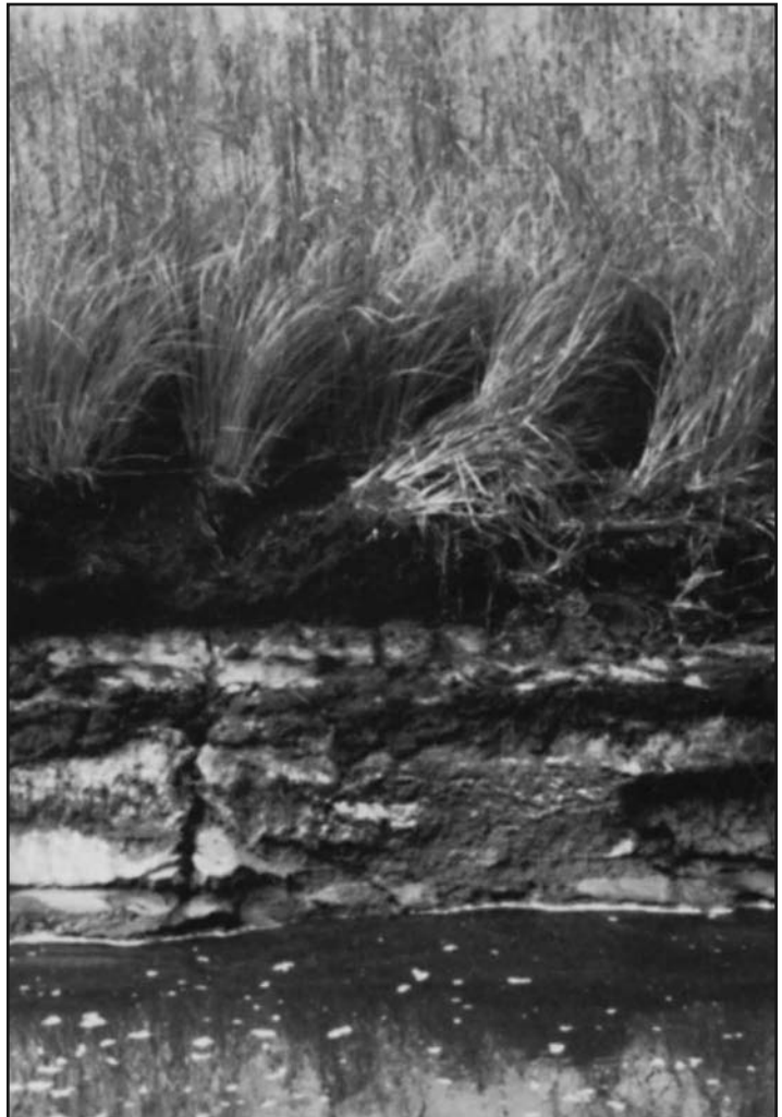
The shallow roots of these upright sedges ( Carex stricta ) are not enough to prevent the organic and silt soils of this streambank from eroding.
